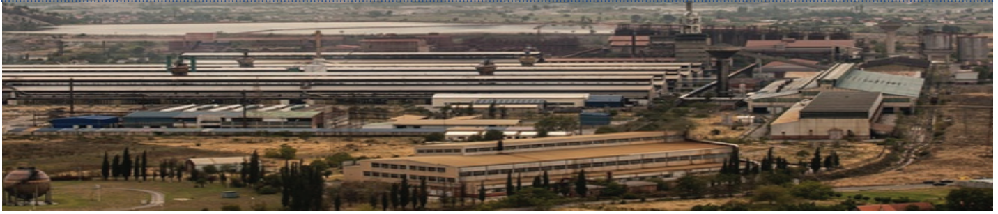
A general view of Montenegro's Kombinat Aluminijuma Podgorica aluminium factory in Podgorica.
