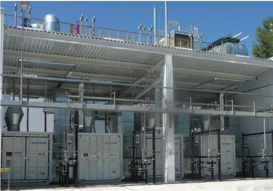
recovery system is that the used hydrogen atmosphere is extracted from the process at lower pressure, while gas purification usually requires a larger pressure differential. Therefore, HyGear's Hy.REC gas recovery technology is based
