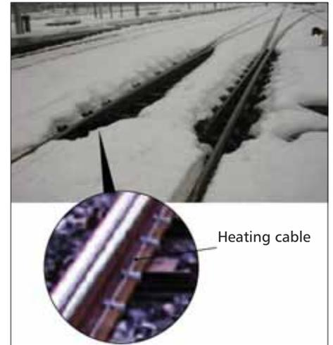
Fig 9 Heating of switch points with aluminium
