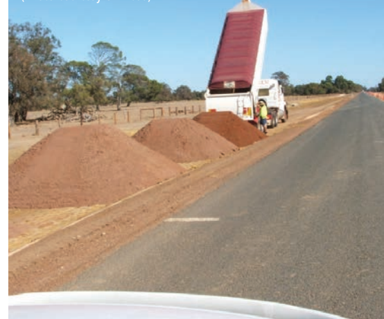
Fig 8. Use of Red Sand™ for road construction (Photo courtesy of Alcoa)
