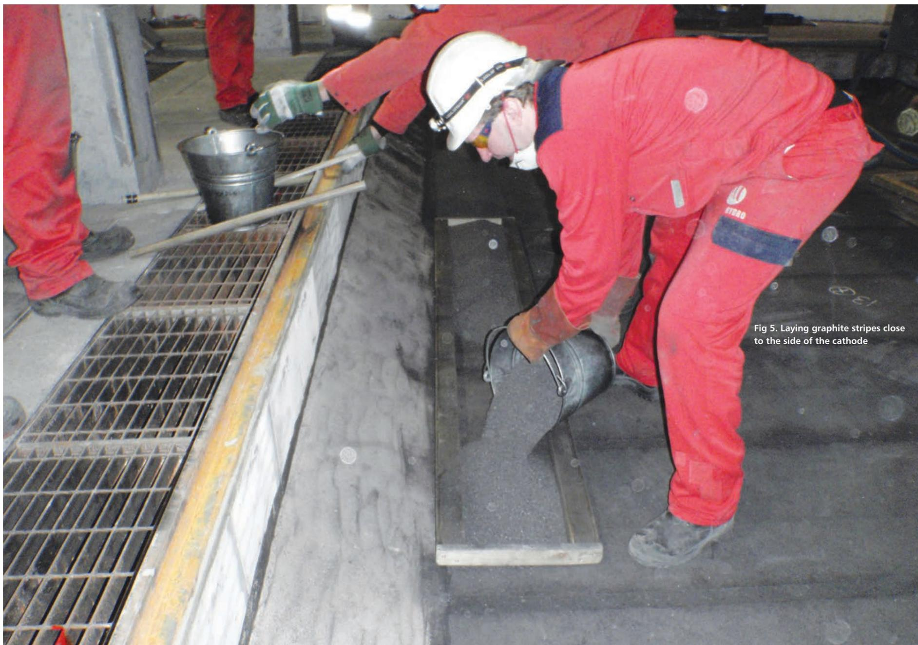
Fig 5. Laying graphite stripes close to the side of the cathode
