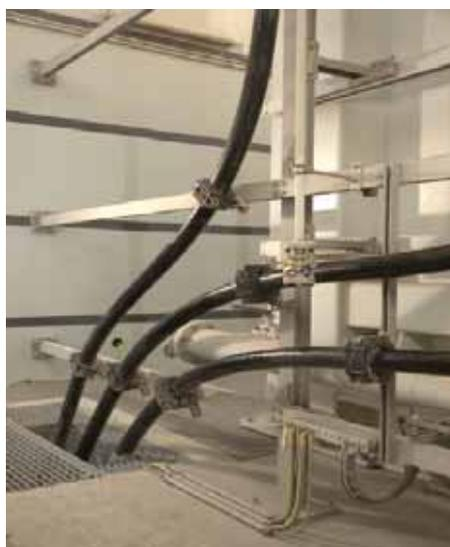
Fig 3 220kV Cable Connection to the Regulation Transformer
