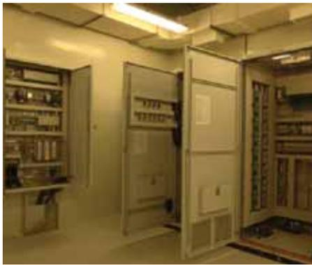
Fig 7 Rectifier control system
