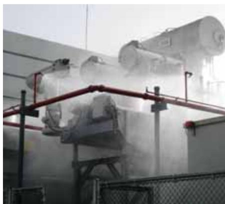
Fig 2 Rectifier bay during fire fighting system testing
