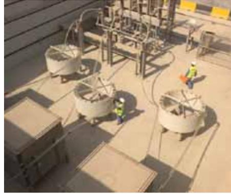
Fig 10 33kV harmonic current filter
